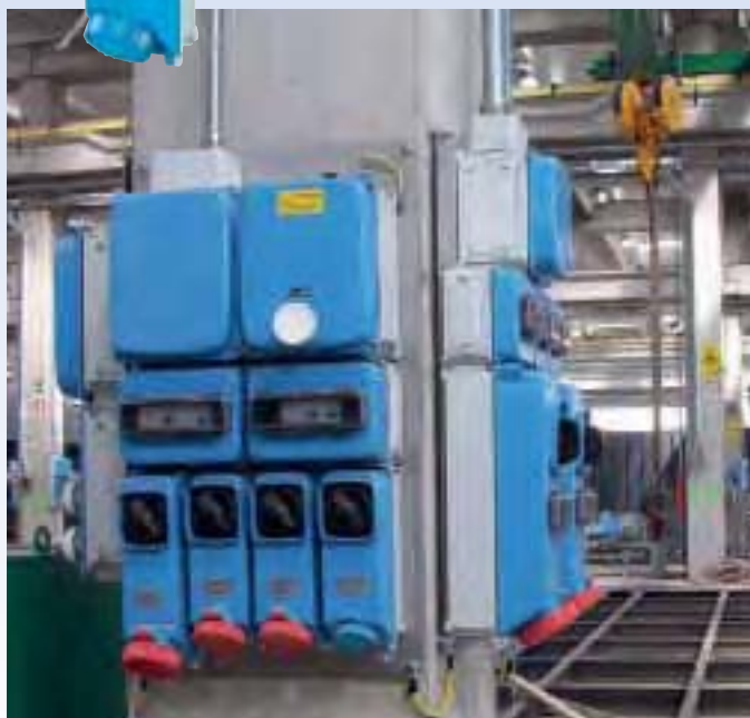
Privilege Building site Civitavecchia
